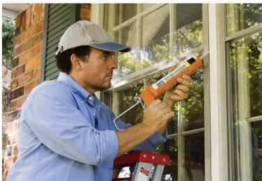
**WINDOW FRAMES.** Use a paintable caulk to seal around the window frames where the interior frame meets the wall. On the exterior, seal around the window where the frame meets the siding. Do not seal
